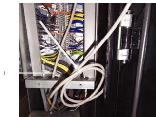
Fig. 32: RJ45 connector
