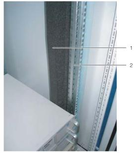
Fig. 16: Foam strip on a server rack upright
