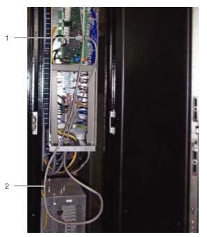
Fig. 33: Connecting RJ45 to pCO Web card
