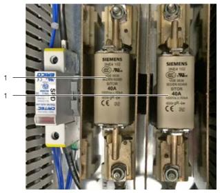
Fig. 27: 40 A Siemens fuses
