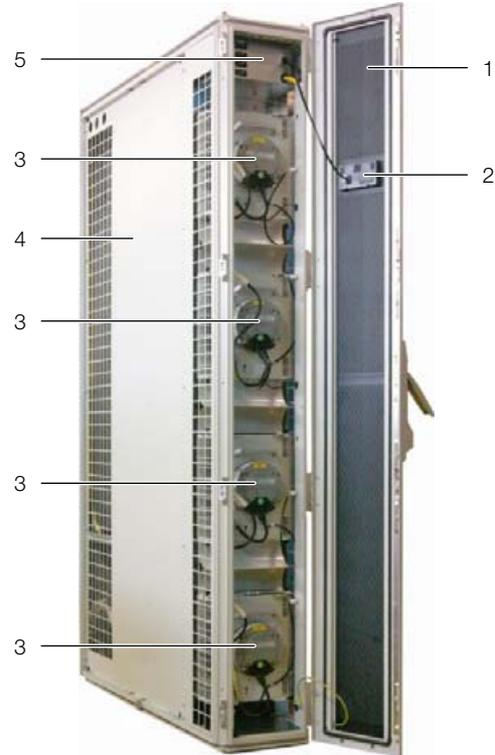
Fig. 7: LCP Rack DX front – open front door
