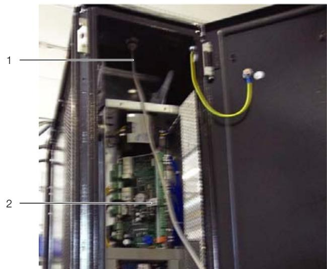
Fig. 30: Installing the pCO Web card
