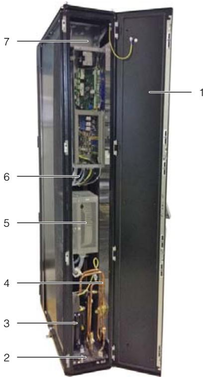
Fig. 8: LCP Rack DX rear – rear door open
