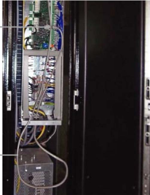
Fig. 33: Connecting RJ45 to pCO Web card
