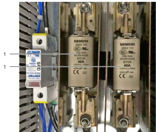
Fig. 27: 40 A Siemens fuses
