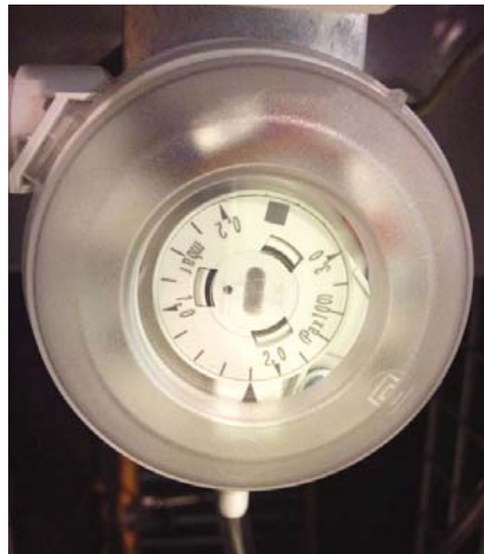
Fig. 59: Adjustment screw at the differential pressure sensor
