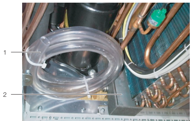
Fig. 25: Condensate discharge
