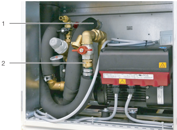
Fig. 23: Connection points at the bottom of the unit
