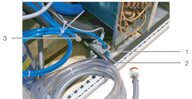
Fig. 63: Connections of the condensate pump
