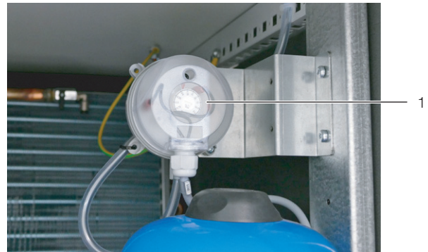
Fig. 64: Adjustment screw at the differential pressure sensor
