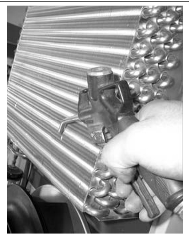
Fig. 30: Clean out the heat exchanger coil and compressor chamber using compressed air
