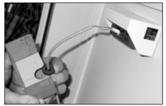
Fig. 16: Insert the cable sleeve
