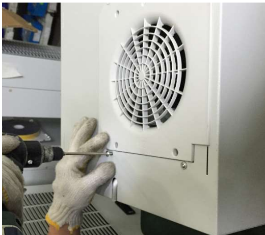
Figure 20: Twist off the screw of the outside fan(2)
