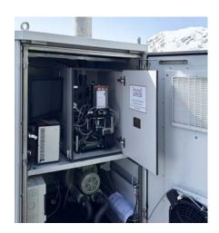
The Toptec boasts a host of valuable features. The enclosure itself and its doors are doubled-walled, preventing heat from penetrating, even in strong sunlight. The double-walled enclosure concept also prevents the formation of condensation. A projecting rain canopy keeps water away from the seal. The Toptec has a high protection category of IP 55 against dust and water jets. This "outdoor enthusiast" is easy-care and robust. It can withstand high winds without damage.
