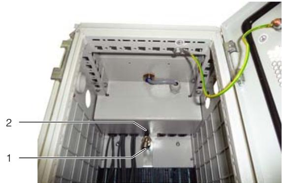
Fig. 47: Bleeding the air from the heat exchanger
