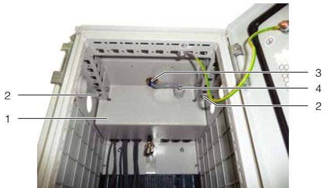
Fig. 38: Access panel removal
