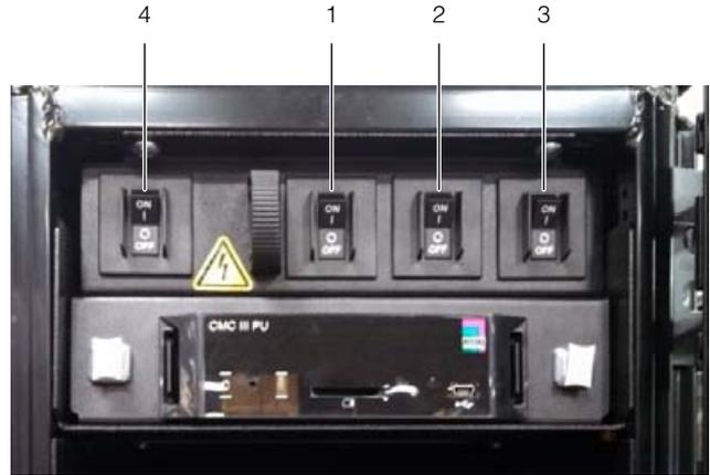
Fig. 13: Fuse box with master switch
