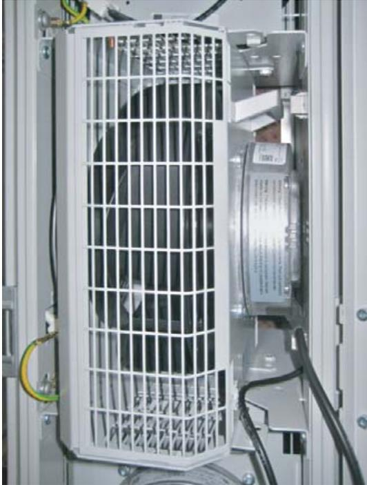
Fig. 30: Rotated fan module in fan tray – LCP Inline and LCP Rack version
