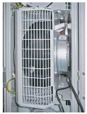
Fig. 30: Rotated fan module in fan tray – LCP Inline and LCP Rack version
