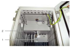
Fig. 47: Bleeding the air from the heat exchanger
