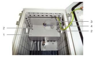
Fig. 38: Access panel removal
