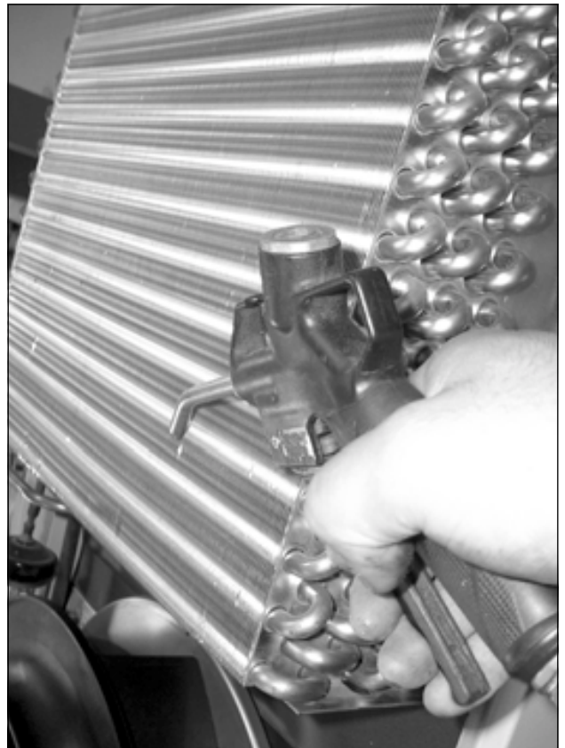
Fig. 58: Clean out the heat exchanger coil and compressor chamber using compressed air (1)
