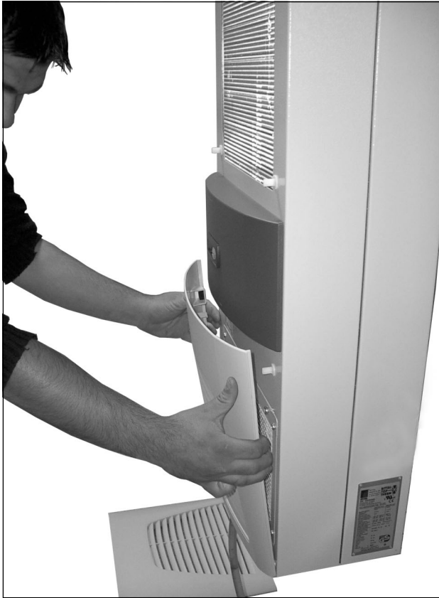
Fig. 43: Remove the lower louvred grille
