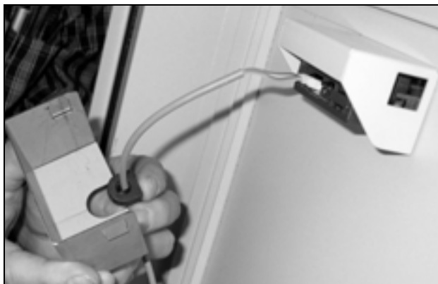
Fig. 16: Insert the cable sleeve
