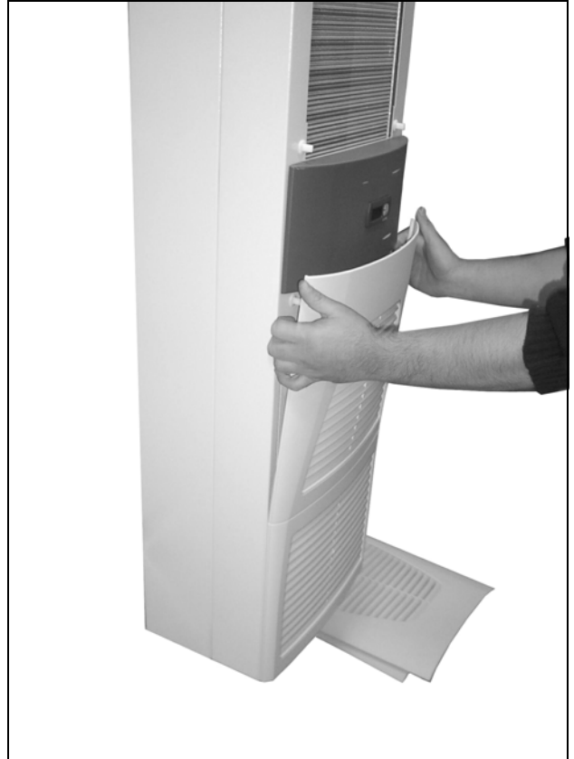
Fig. 57: Remove the bottom louvred grille (1)
