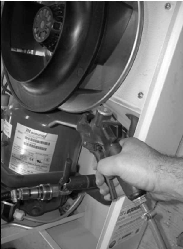
Fig. 76: Clean the heat exchanger coil and compressor chamber using compressed air (3)
