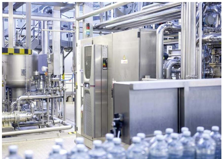
While the bottles rattle by, the Rittal Blue e+ cooling units reliably do their job – despite the significant seasonal temperature fluctuations that can occur in the bottling plant.
