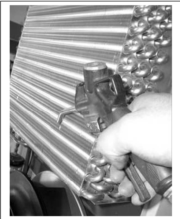
Fig. 27: Clean out the heat exchanger coil and compressor chamber using compressed air
