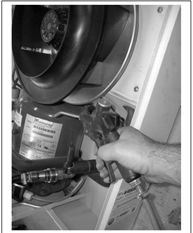
Fig. 28: Clean out the heat exchanger coil and compressor chamber using compressed air
