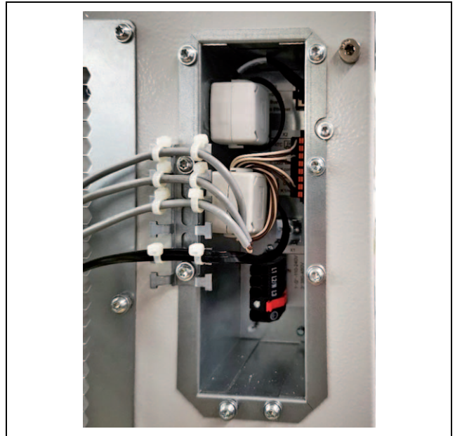
Fig. 33: Mounting point for the ferrite cores on SK 3486330, SK 3487330, SK 3488340, SK 3489340
