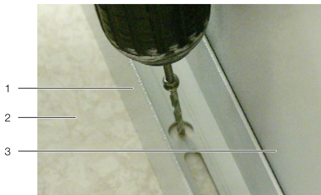
Fig. 8: Drilling the fastening holes
