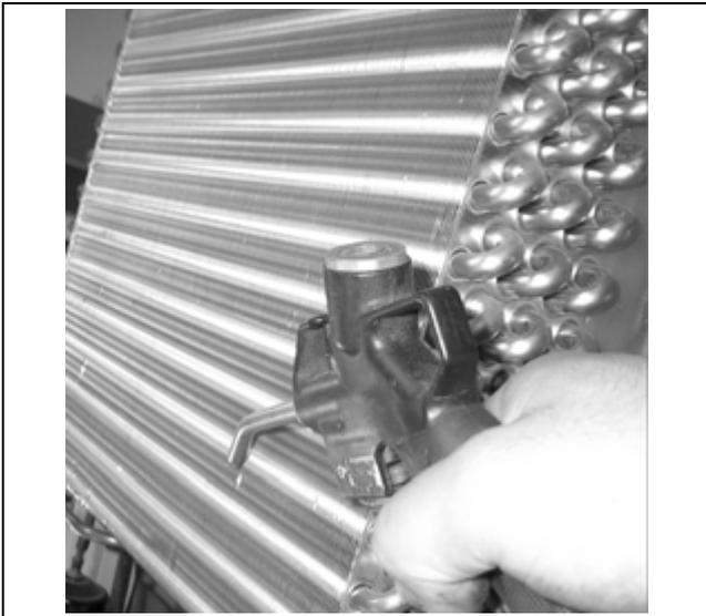
Fig. 47: Cleaning the condenser
