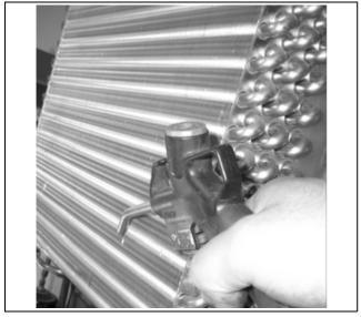
Fig. 47: Cleaning the condenser
