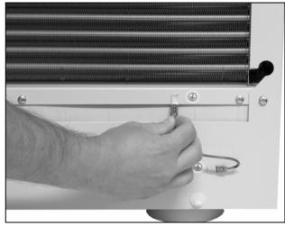
Fig. 25: Disconnect the earthing cable
