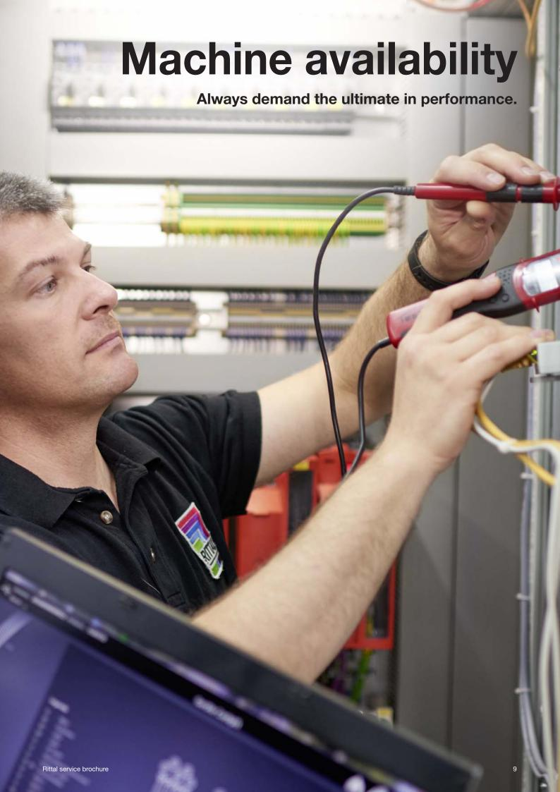
Fault-free operation of production lines depends to a great extent on the heat load to which the individual electronic components are subjected. An increase in temperature of around 10 K (Kelvin) halves the service life of these components and doubles their failure rates.
