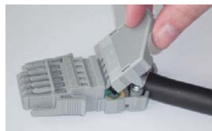
Fig. 65: Closing the strain relief housing
