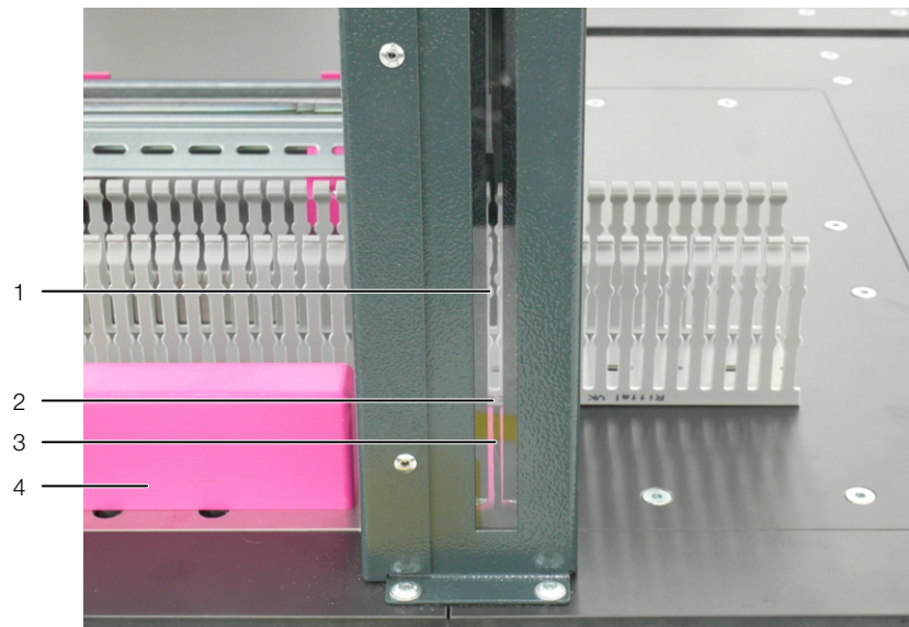
Fig. 13: Alignment of a cable duct
