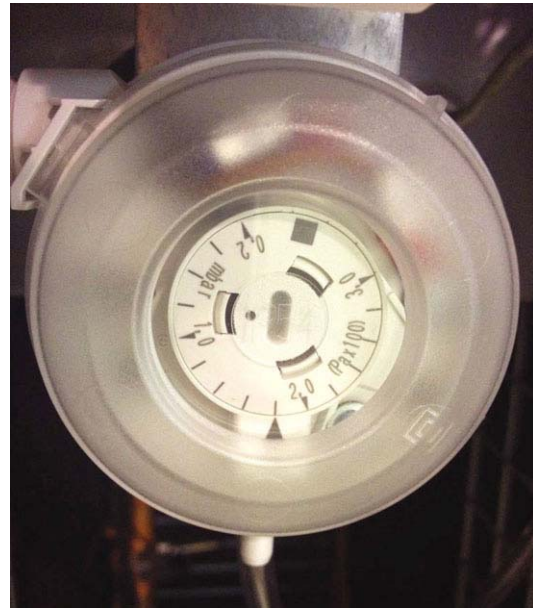
Fig. 62: Adjustment screw at the differential pressure sensor
