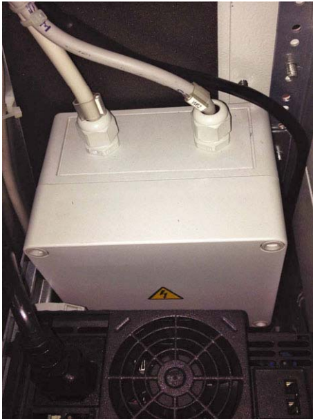
Fig. 57: Additional box for the thermal protection of the electrical heaters
