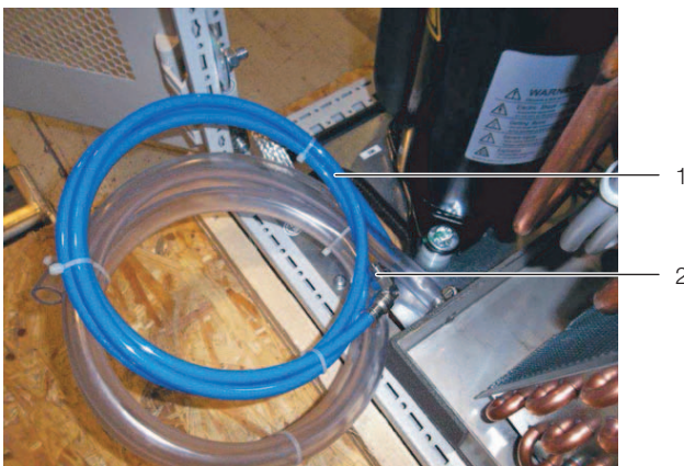
Fig. 53: Connection hose with 1/8" external thread adapter
