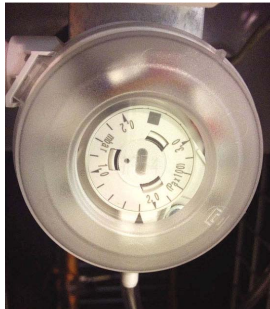
Fig. 60: Adjustment screw at the differential pressure sensor
