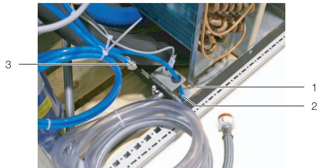
Fig. 64: Connections of the condensate pump
