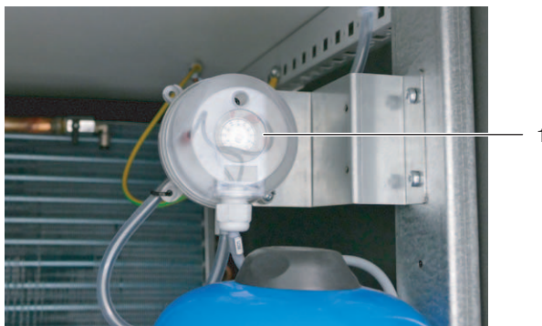
Fig. 65: Adjustment screw at the differential pressure sensor
