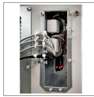
Fig. 33: Mounting point for the ferrite cores on SK 3186330, SK 3187330, SK 3188340, SK 3189340
