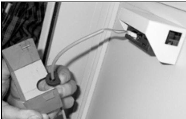
Fig. 16: Insert the cable sleeve
