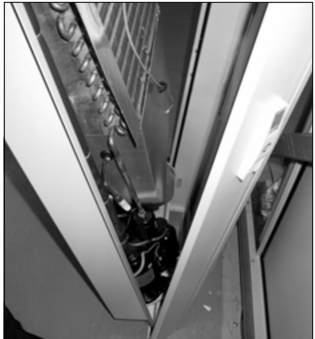
Fig. 8: Fit the climate control module in the section door
