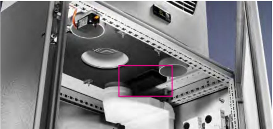
These use an efficient PTC heating cartridge with automatic adjustment of thermal output depending on the amount of condensation. Approx. 120 ml of condensate can be evaporated per hour. This ensures complete removal of condensate.
