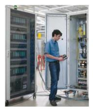
inspection. Checks must be carried out to ensure that all measures for compliance with the designated degree of protection have been implemented. The routine verification contains the individual verification, the test specification, the test result, the name of the person performing the test, and the documentation date.
