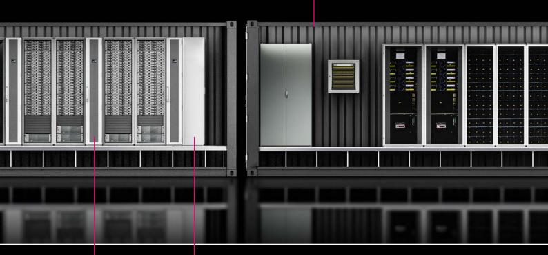
Low-voltage distributor: Complete distributor system with connection point for the main supply and the outgoing feeders from all PDUs
