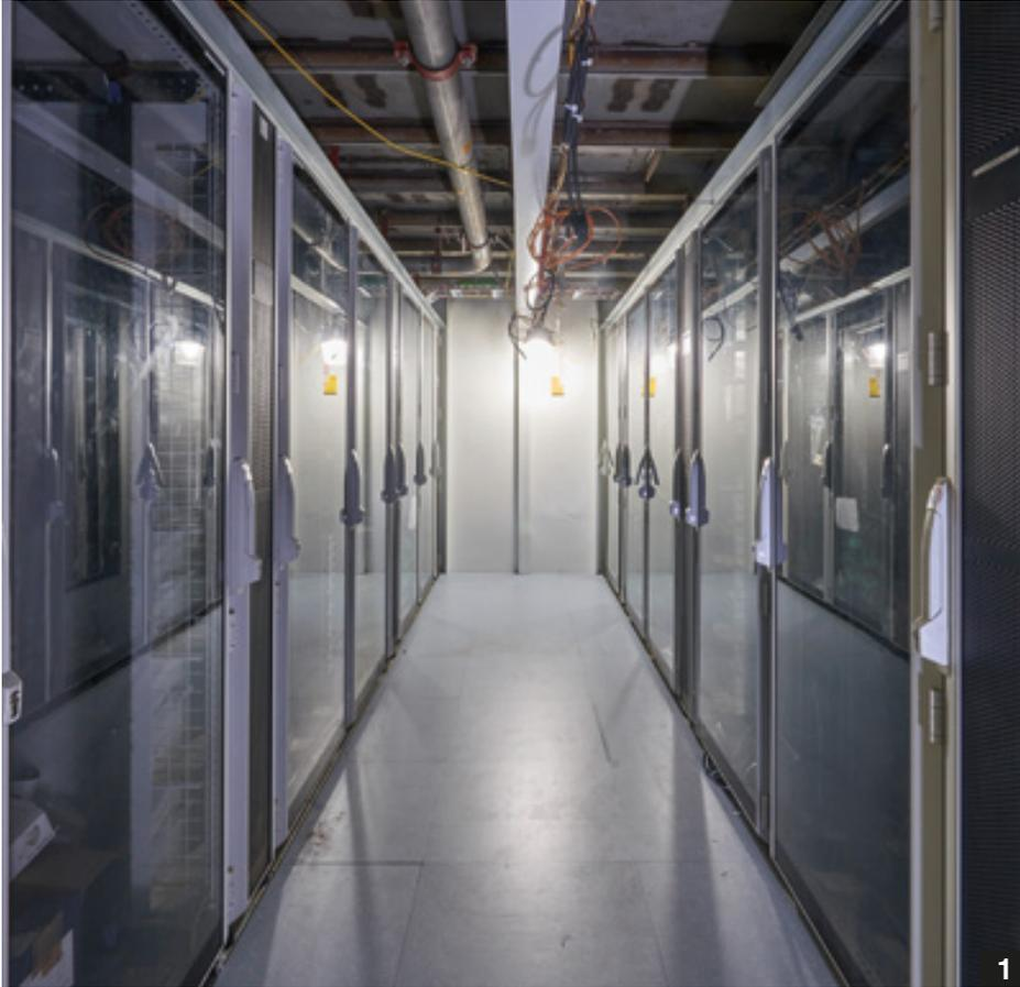
1) Two redundant data centers are located in different fire zones on board. The picture is from the construction phase.
