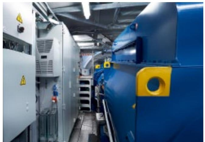
Converters in the nacelle are securely accommodated in TS 8 enclosures from Rittal. These enclosures are also spring-mounted on rubber bearings and steel beams at the top and the bottom due to the constant movements and vibrations.
