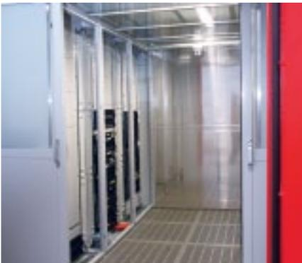
Cold-aisle containment in the data centre of Vitos Haina gem. GmbH reliably prevents hot and cold air mixing.
