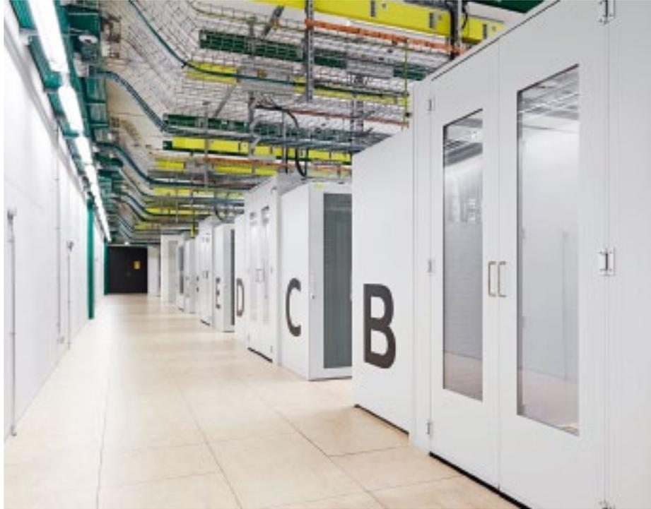
On completion of all four modules, the data centre will have 600 racks. With a good 25,000 U, it can accommodate around 6,000 servers and network components.
