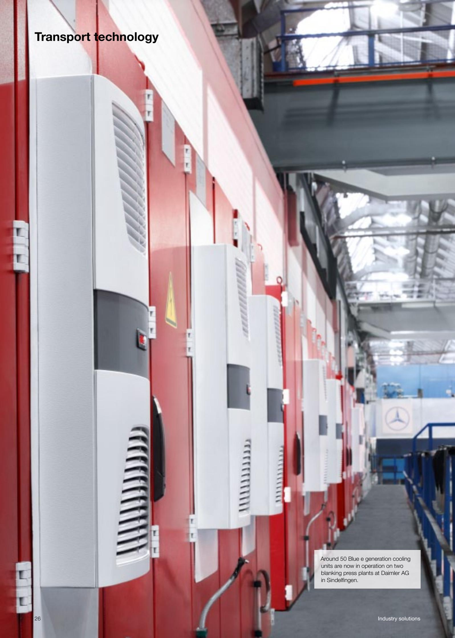
Around 50 Blue e generation cooling units are now in operation on two blanking press plants at Daimler AG in Sindelfingen.
