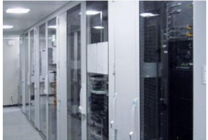
To stop it getting too warm in the narrow confines of the computer rooms on the luxury liner, the operator decided to air-condition the server racks directly using liquid cooling packages from Rittal.
