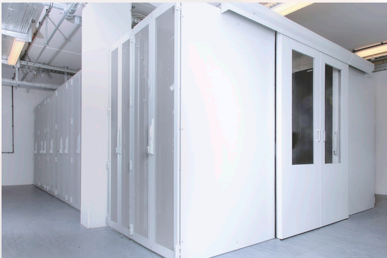
The Manner servers are accommodated in 14 Rittal TS IT racks, which are arranged in two rows facing one another to form the cold aisle.
