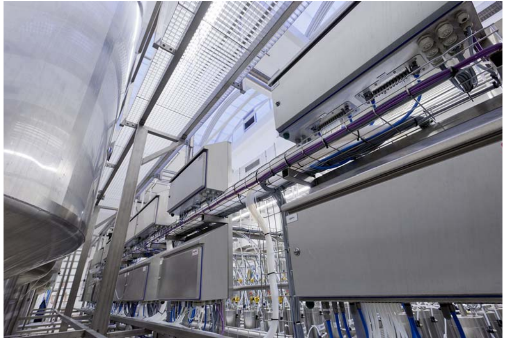
Figure 2: Automation technology at FrieslandCampina is safely protected by Hygienic Design enclosures from Rittal.
