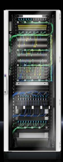
Let innovative hybrid technology take the energy efficiency of your rack cooling to a whole new level. An active cooling circuit with speed-controlled components provides demand-based cooling. As soon as the ambient temperature drops below the set level, the integral heat pipe takes over climate control of the rack with passive cooling. This will unlock huge energy savings.
