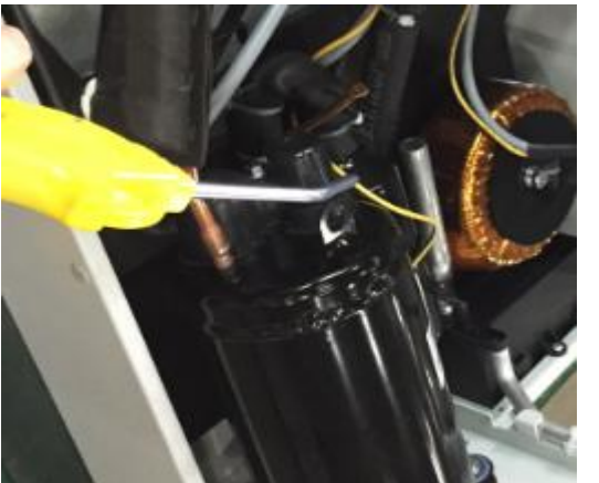
Figure 24: Clean the heat pipe and compressor chamber using compressed air
